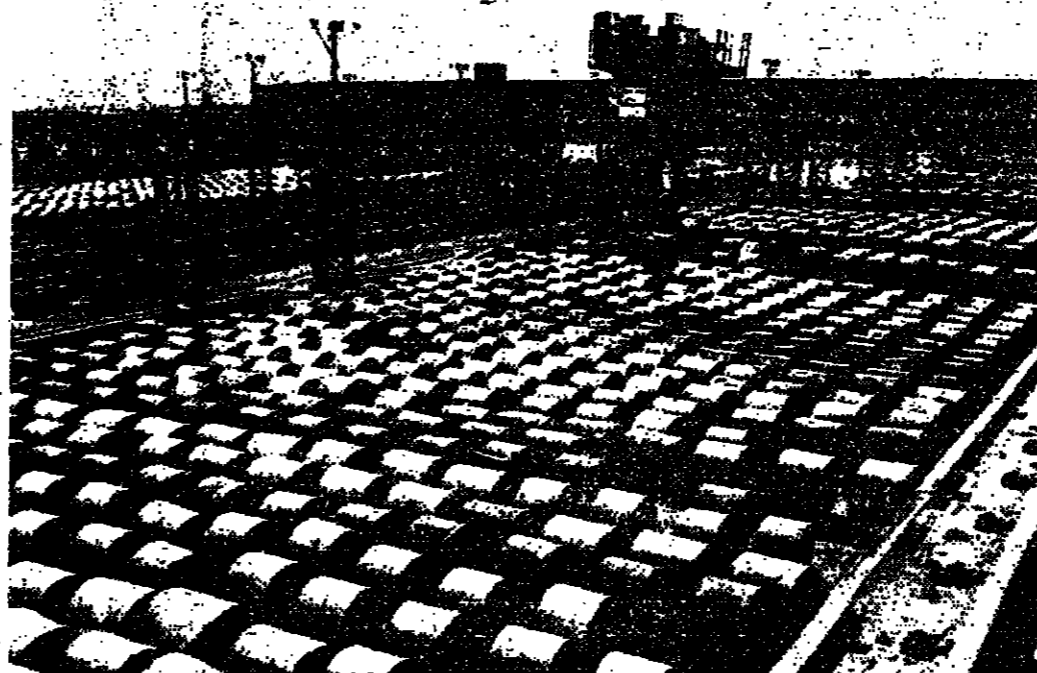
Coil stockyard at Shotton Works
